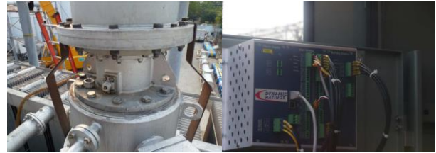
Figure 3. Test/Potential tap of bushing and installed DTM-6.
