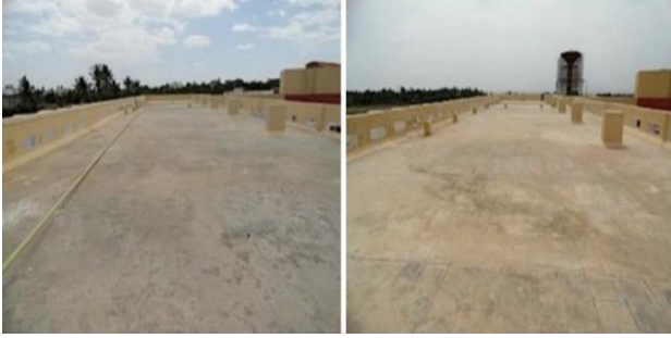
Figure 4. Roof of department building
